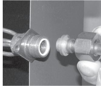
II-4. Slide the 13/16" nut over the lineset and separate the two halves of the flowrator.
