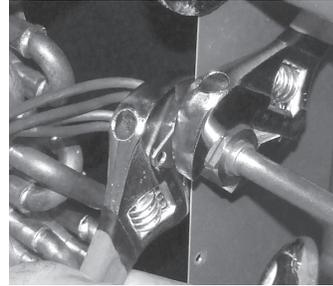
II-3. After ensuring that the coil is free of any residual pressure, disassemble the flowrator body completely using two wrenches. Take great care not to distort the feeder tubes. The wrench used to clasp the nut should be turned in counter-clockwise direction to unscrew the nut.
