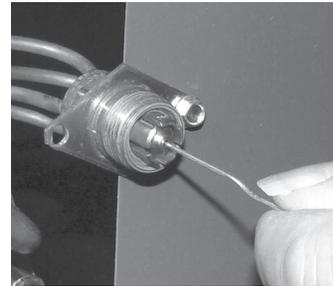
II-5. Pull the piston out using a small wire or pick. Verify the piston size (size is typically stamped on the body of the piston - Fig 7A-2). If a different piston size is required by the outdoor unit manufacturer, replace the piston using the small wire provided with the piston kit.
