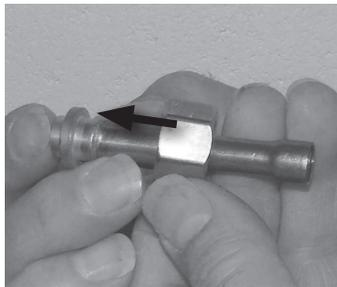
I-3. Slide the attachment nut onto the liquid line stub out.
